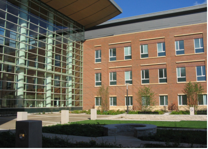
Business Instructional Facility (BIF) courtyard. Glass wall facing South
