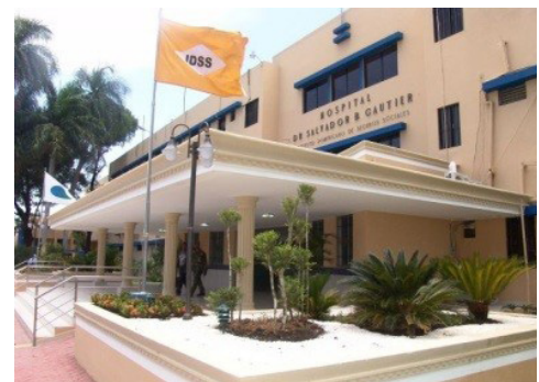
Hospital Dr. Salvador B. Gautier, Santo Domingo, Dominican Republic. Photo credit: Richard Bido-Medina
